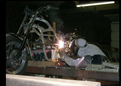
Welding the battery racks at Taylor's Portable Welding
